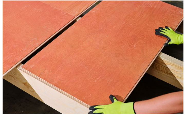
Fig. 7: Installation of plywood panels on a roof structure.
